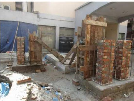
Shuttering work of RC-jacketing for brick column
