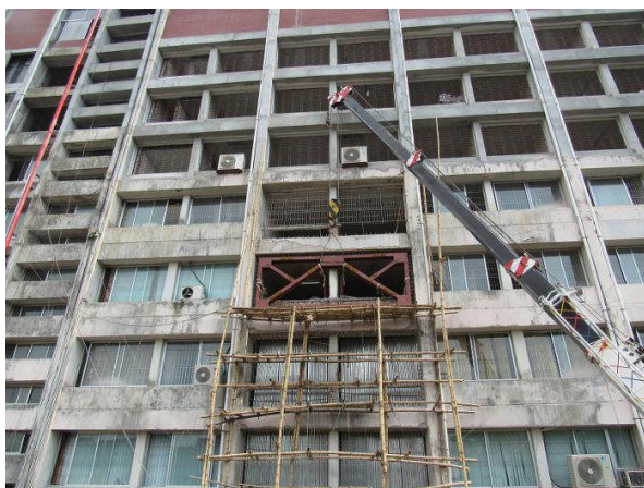
Installation of brace at high levels
